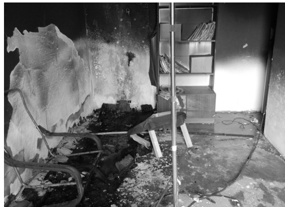
Fig. 6 Fire compartment after test no.2
