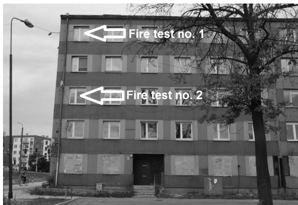
Fig. 1 External view of the building
