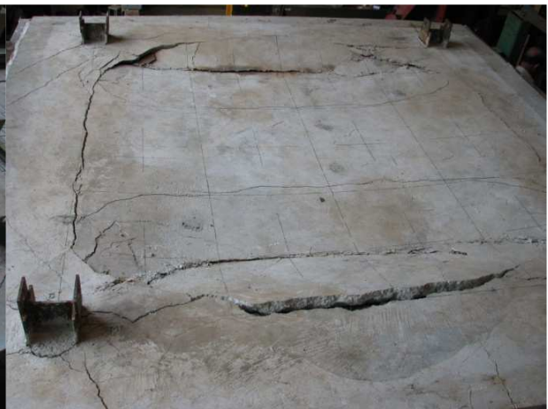
Fig. 7 Crack pattern of S3-FR
