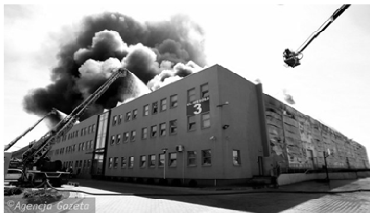
Fig. 1 View of the complex during the firefighting (internet source); in the foreground the administrative-office part of the building is seen
